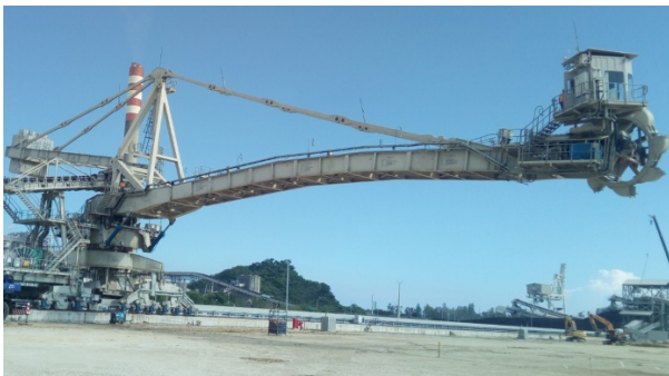
Figure 1. Stacker-Reclaimer at the coal yard
