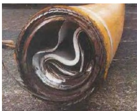
Figure 2. Collapse failure of the flexible riser [7]
