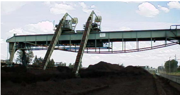
Figure 1 – Bridge-type stacker-reclaimer; Power plant “Kolubara” – Veliki Crljeni
