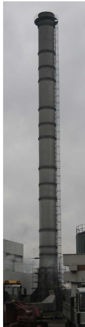
**Figure 1. Industrial steel chimney of auxiliary boiler facility in TENT 'B' power plant**
