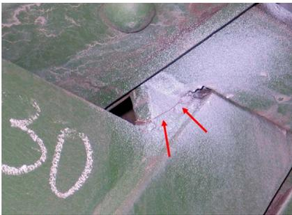
**Figure 9. Crack of the gusset plate resulting from a notch caused by a step change in stiffness**
