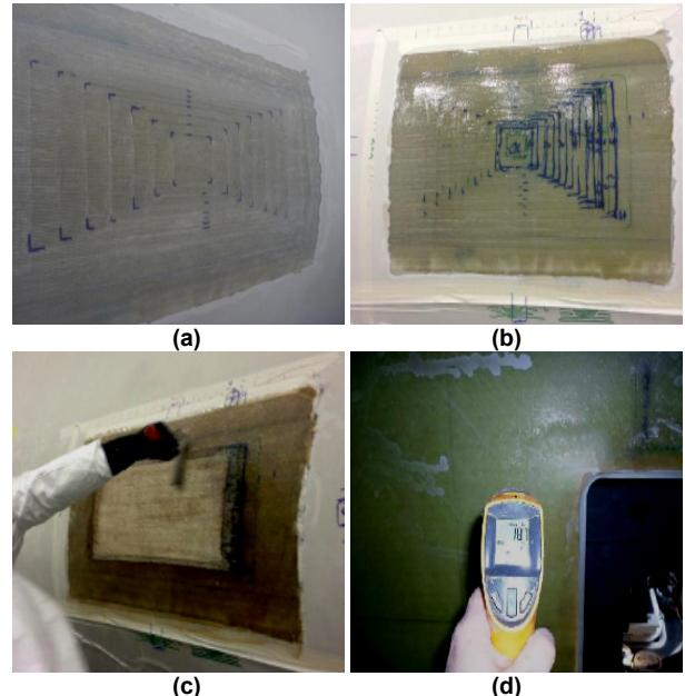
**Figure 11.** Repair process involving, (a) grinding and chamfering of damaged area, (b) application of resin layer, (c) hard roller to roll out each layer and remove excess resin and (d) temperature measurements before and after repair.
