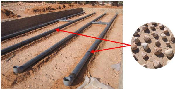
**Figure 2. PVC tubes in H-shape filled with rocks**
